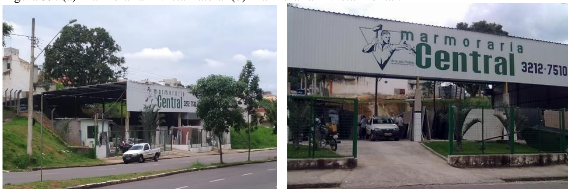
Figura 59: (a) Marmoraria – Vista Lateral (b) Marmoraria – Vista Frontal.
