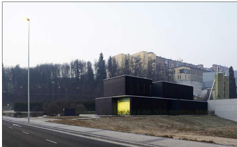
Figura 23: Vista Frontal Shelter Home.
