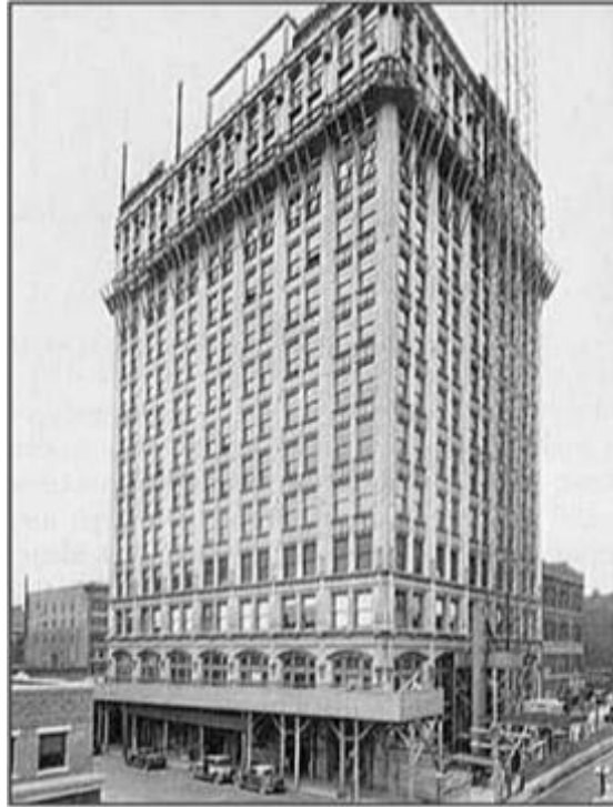
Figura 5: Edifício Southwestern Bell Telephone Company.
