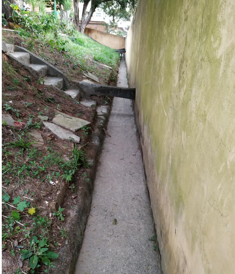
Figura 9 - Conductor de concreto
