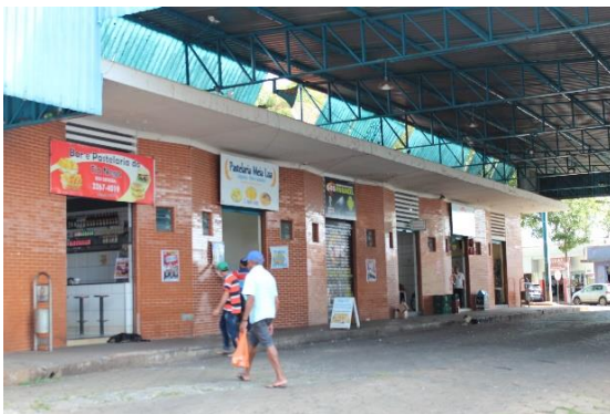
a) Fachada principal
